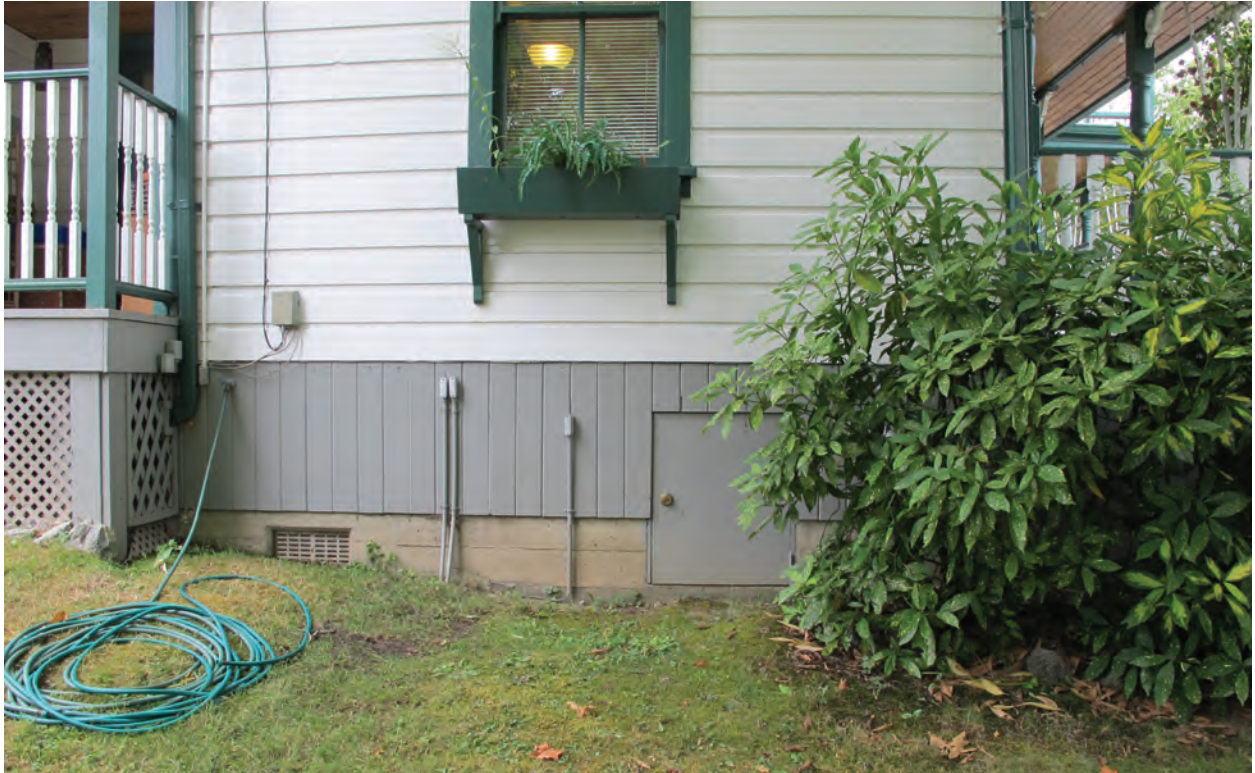
Vertical tongue-and-groove cladding and exposed poured-in-place concrete foundation below
