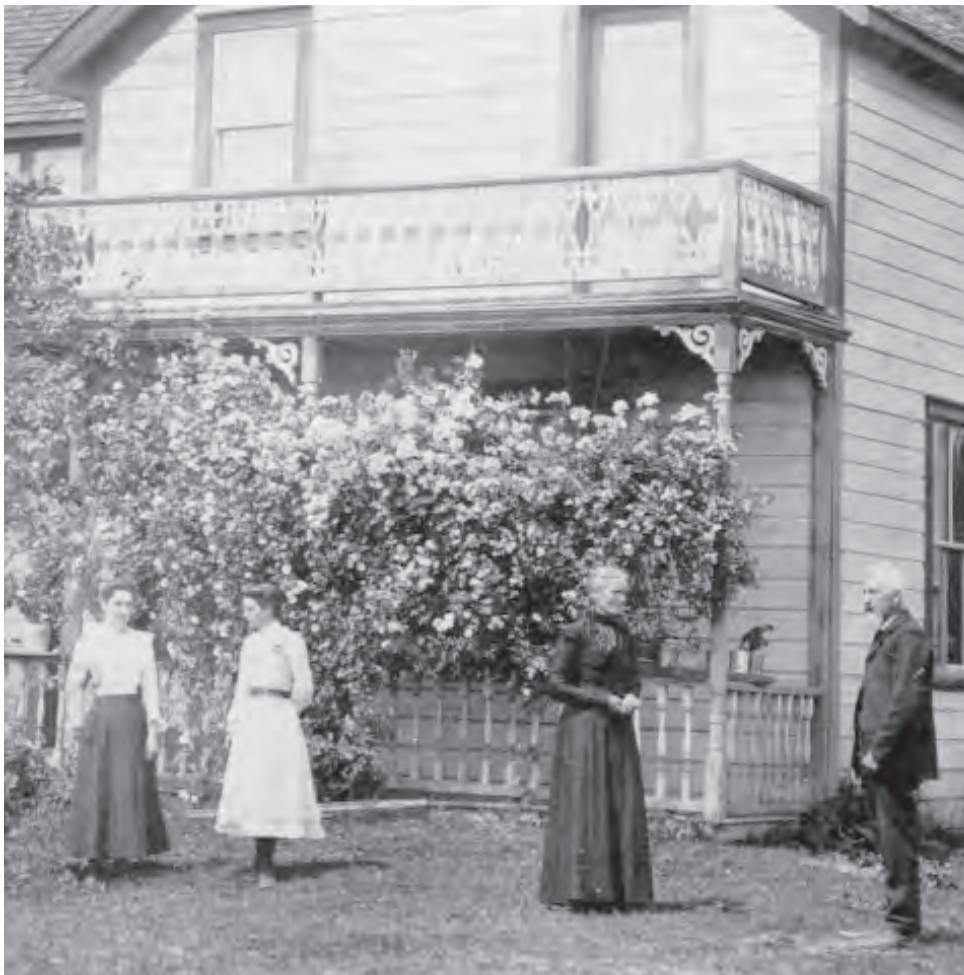
Archival images showing the earliest recorded appearance of the front verandah and balcony. Note the difference in balustrade height and details, as well as the column profile and colours.
