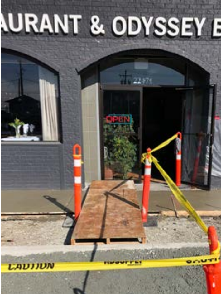
New temporary ramp leading to businesses during concrete sidewalk pour.
