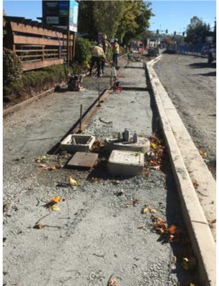
Preparation for sidewalk pour on the north side of Lougheed Highway
