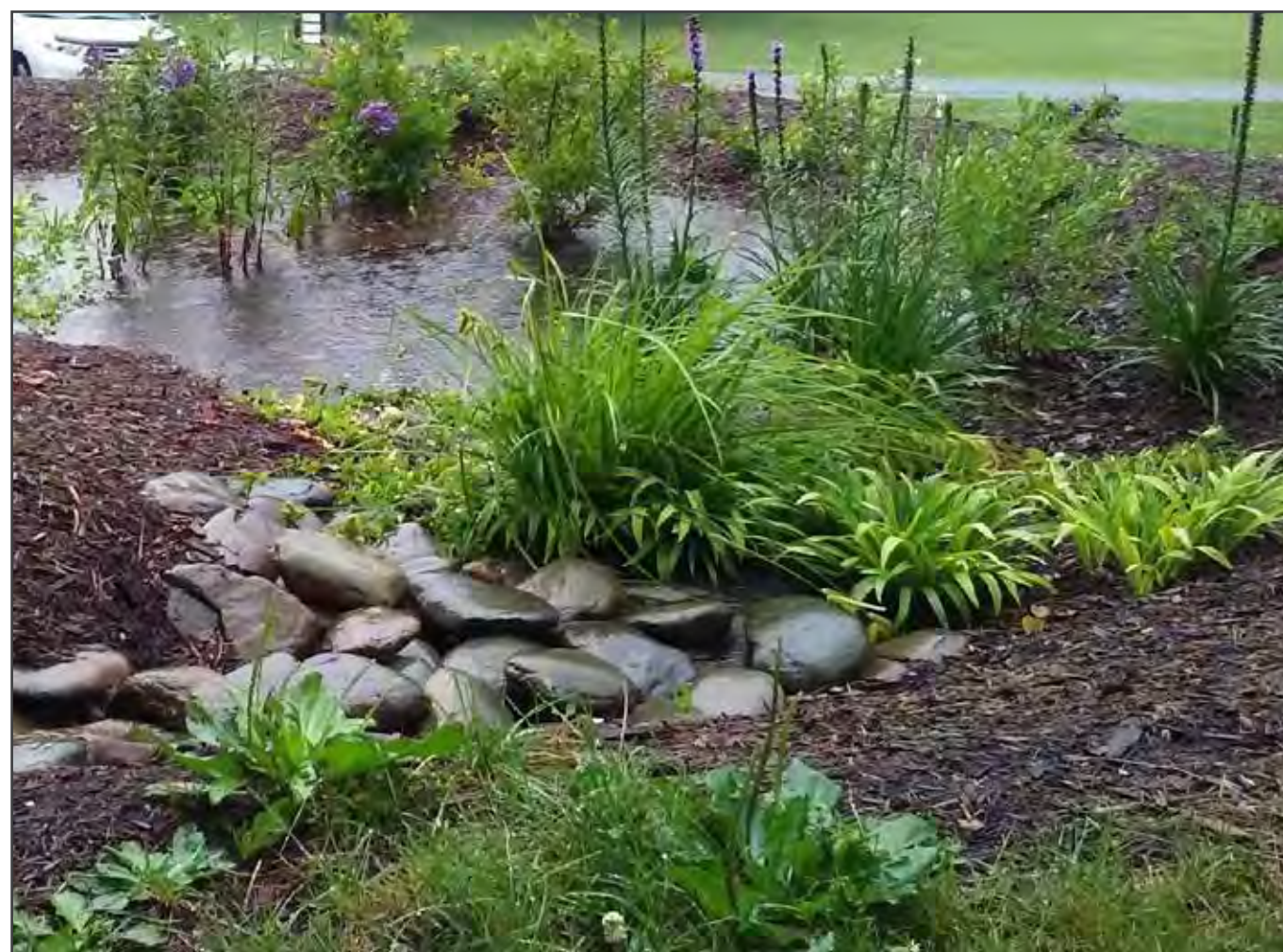
Image: Stormwater Pond and Biofiltration Feature
