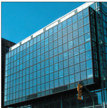
Figure 1: PV's integrated into the glass of classroom walls at Red River College's new Princess St. Campus in Winnipeg.
