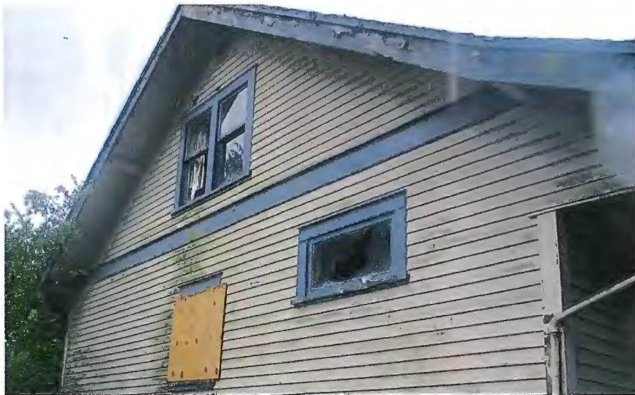
Gillespie Residence Side Elevation Windows Partially Intact. Overall Sashes and Jambs.
