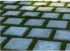
Figure 127: Permeable pavers minimize imperviousness
