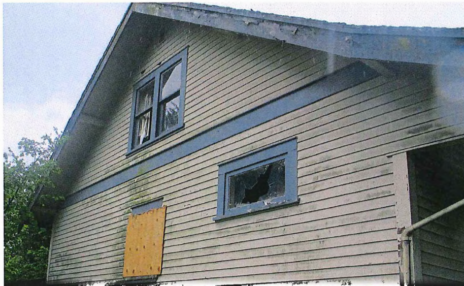
Gillespie Residence Side Elevation Windows Partially Intact. Overall Sashes and Jambs.
