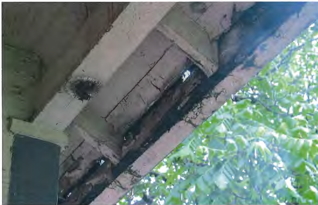
Gillespie Residence Front Entrance Rot Condition At Soffit and Trim Board Interface.
