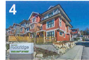
3 STOREY TOWNHOUSE DEVELOPMENT MATERIALS: BOARD & BATTEN, HORIZONTAL SIDING & SHAKES
