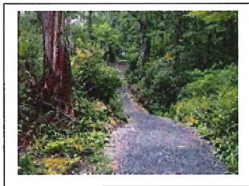
Trail with 2.5 metre with and 250 mm shoulder
