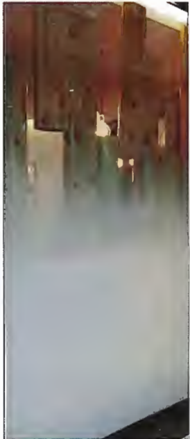
ombre effect opaque window film on storefront glazing (transparent section at top of window only, no sightlines into store)
