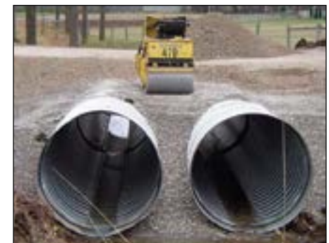
Image: Storm sewer pipes example
