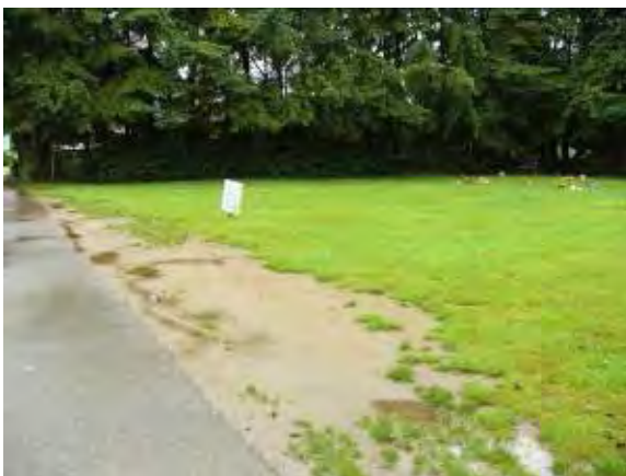
Erosion issues caused by cars driving over turf
