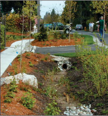
Figure 10: Rain garden / infiltration swale
