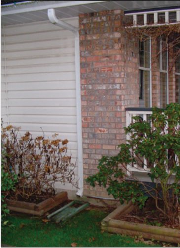
Figure 9: Disconnected downspout
