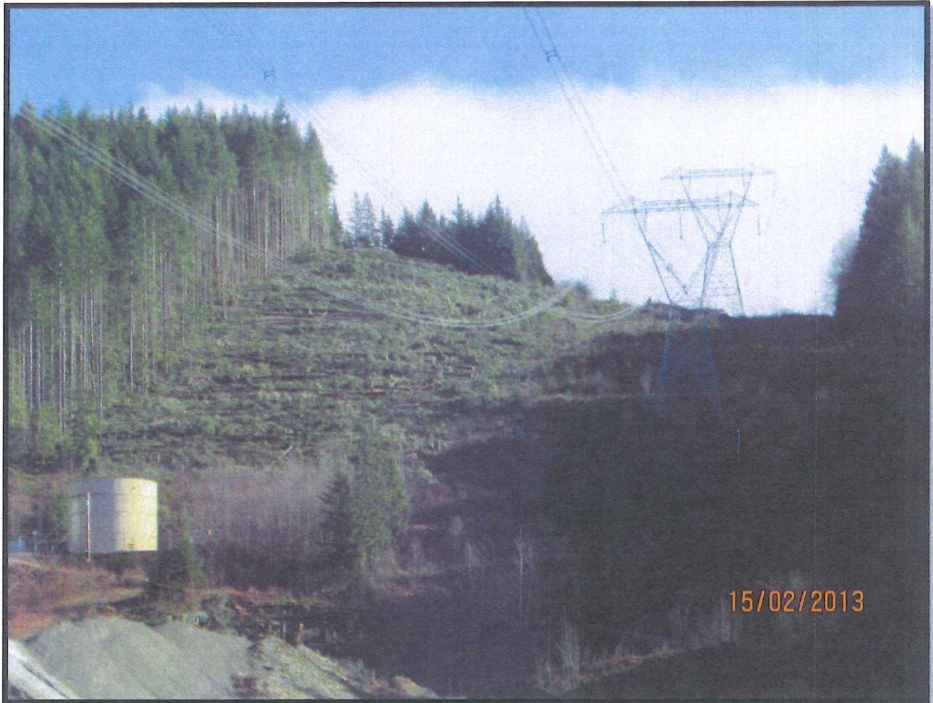
Figure 8 Recent tree falling for BC Hydro transmission line twinning project – potential community fuel break or short-term fuel hazard depending on proposed vegetation management regime. This highlights the need for inter-agency communication and collaboration.
