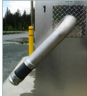
*75 mm (3 inch) male cam-lock fitting from filling station to female
