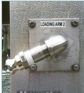
*25 mm (1 inch) male cam-lock fitting from filling station to female
