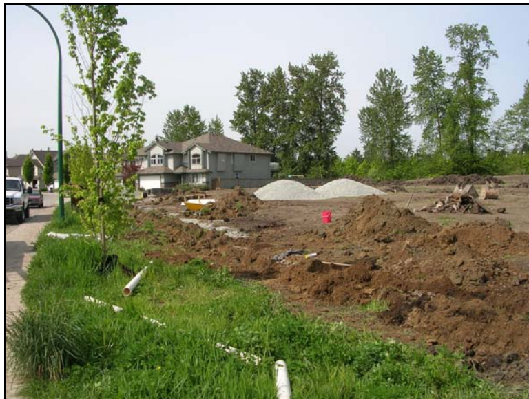
Boundary Park Construction
