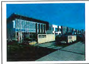
Signage should complement building design and placement
