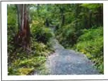
Trail with 2.5 metre width and 250 mm shoulder
