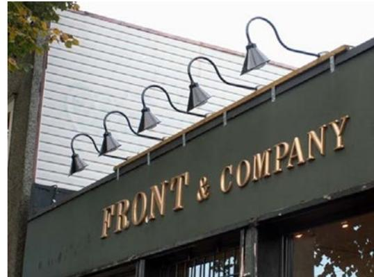
*Figure 47: Gooseneck lighting highlights signage and directs light.*
