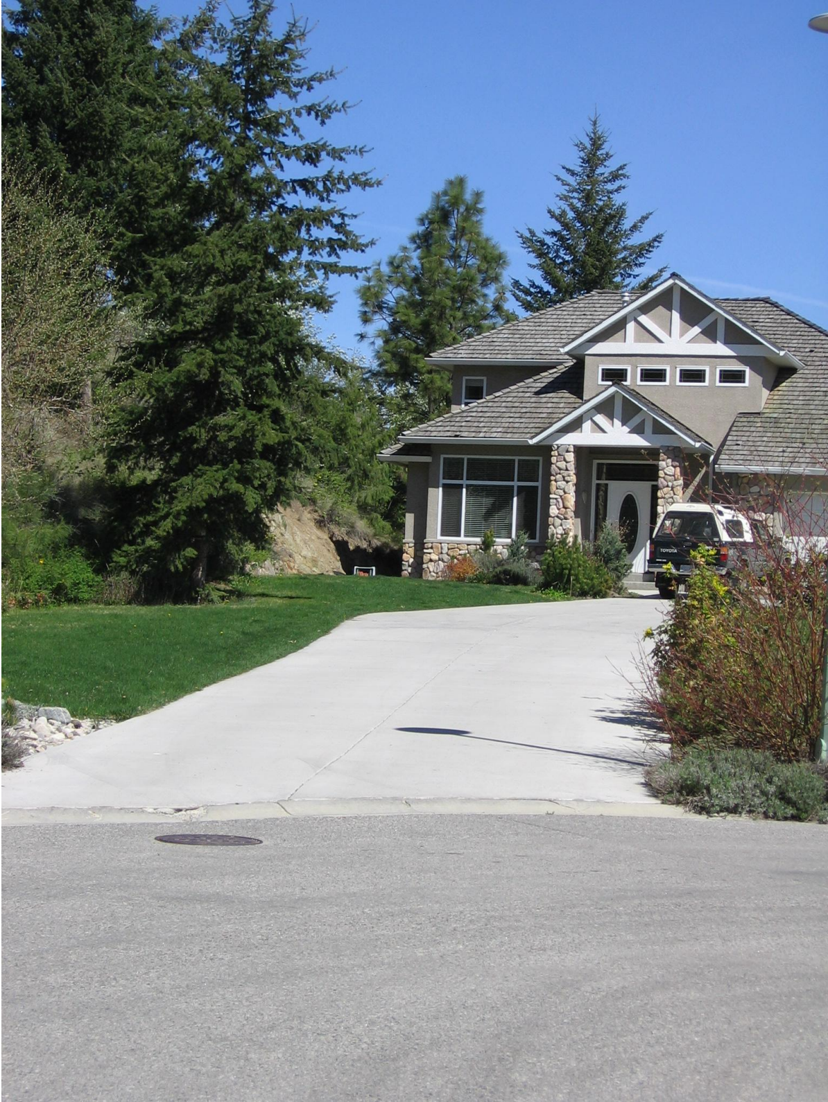
Figure 18. Photograph showing unrated roofing material present on many homes within the District wildland urban interface.
