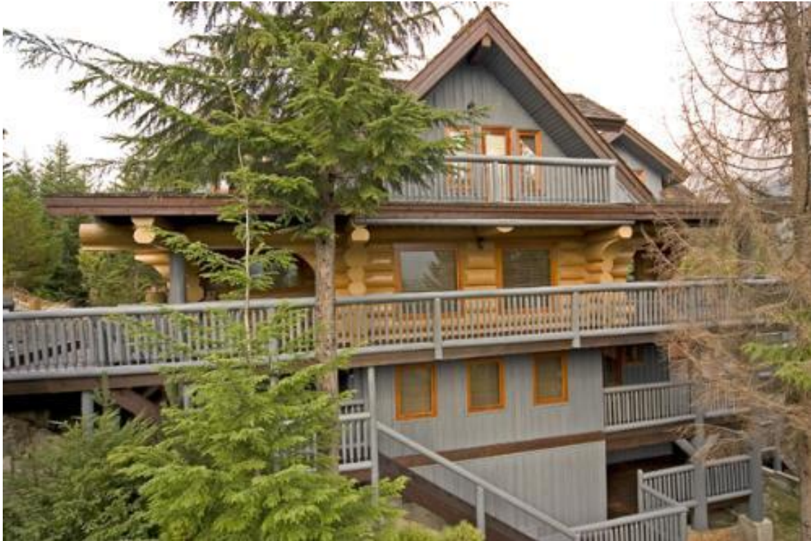
Figure 19. Example of home with wood siding and open decks and balconies.
