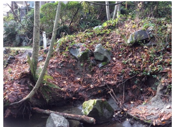
Photo A-2: Bank Erosion @ River Rd. near River Bend Facing Southwest
