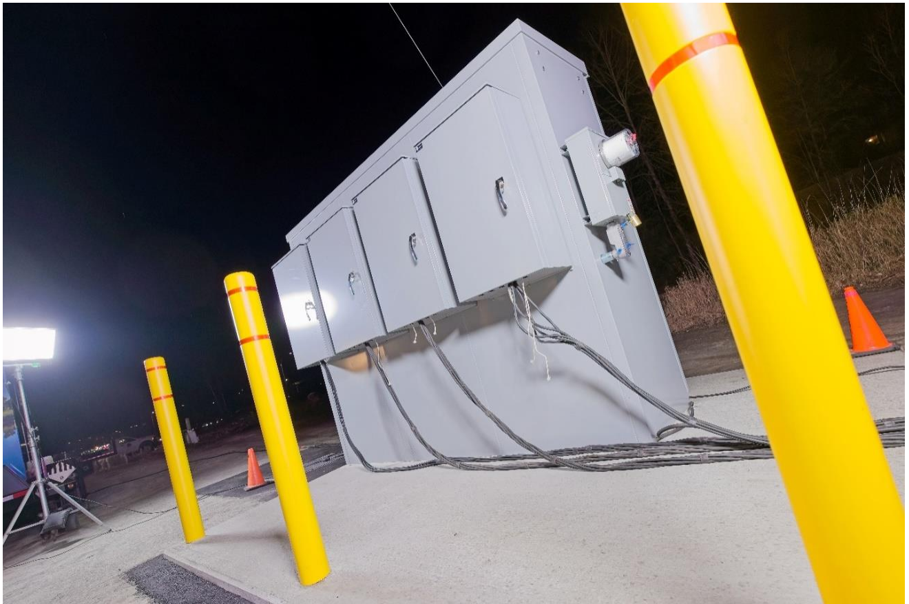
Figure 8: Completed Kiosk at the Railway lot
